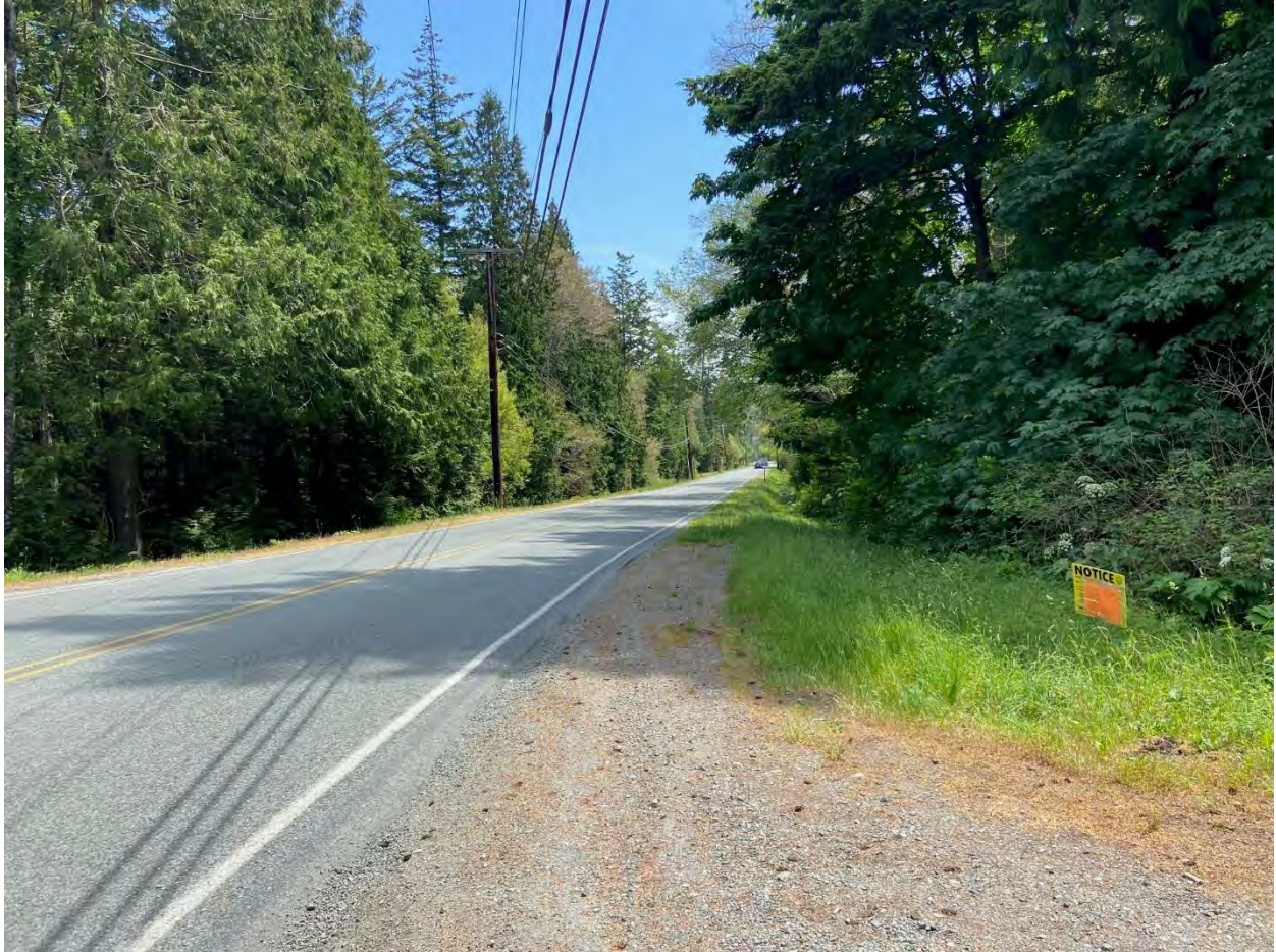
Rosario Road, Looking east/southeast
